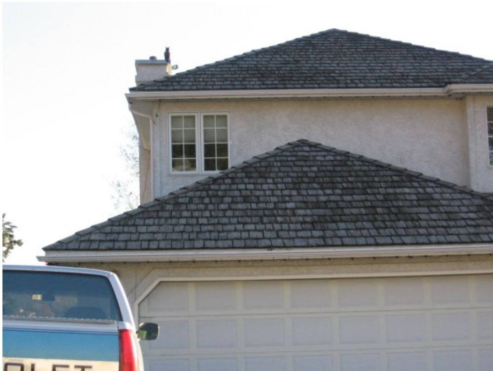
Figure 2. Photograph showing a wood shake roof.
